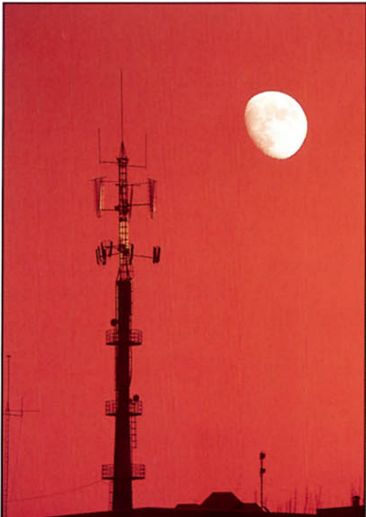
Digital exchange aerial at Albéniz (Madrid)
