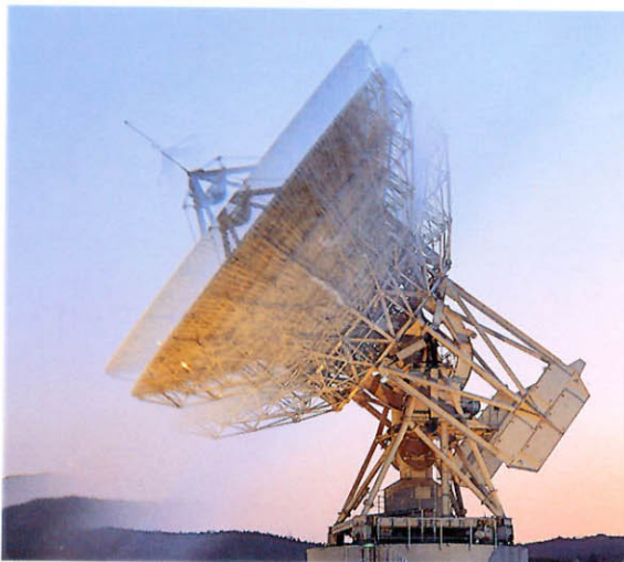
The Telefónica Group companies use an infrastructure which is constantly being upgraded. Armuña de Tajuña Satellite Communications Centre Antenna
