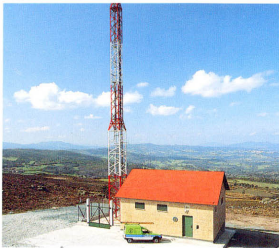
Cellular access rural telephone antenna in Galicia
