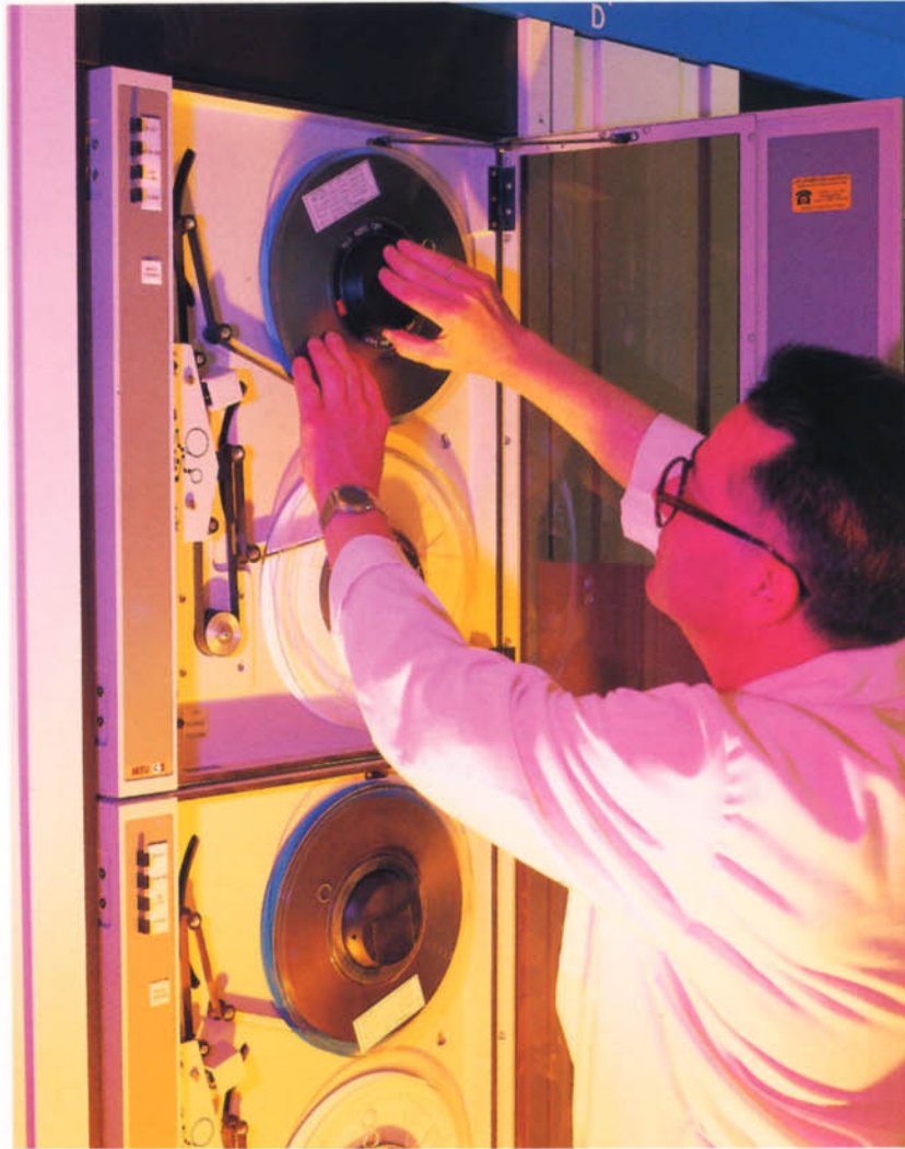
Inspection work at the Cartuja-Sevilla digital exchange.
