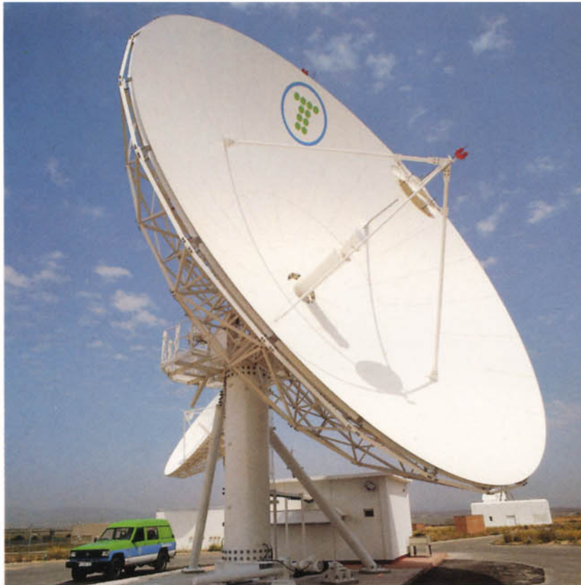
Detail of the Penedés Satellite Communications complex.
