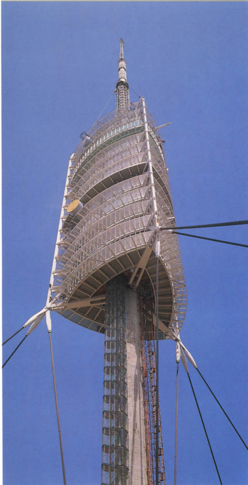
Detail of the Collserola Communications Tower, Barcelona.
